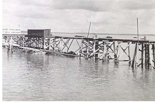
This photo is of a temporary refuelling position constructed on the hull of S.S. "NEPTUNIA" which was sunk during the 19 Feb 42 Japanese air attack.
